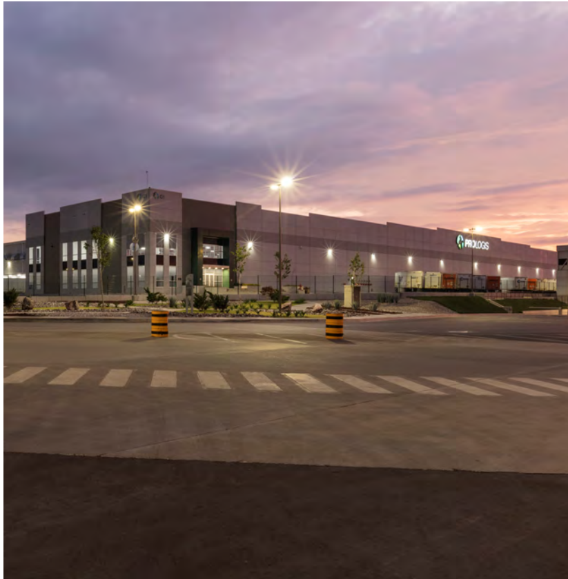
Park Grande, Building 1, Mexico
