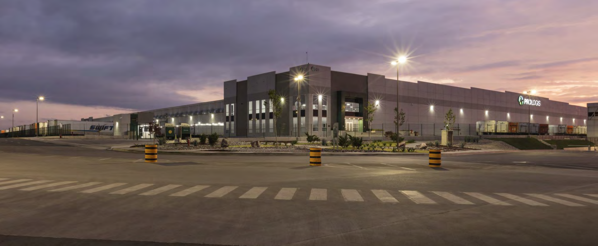
Park Grande Building #1, Mexico City, Mexico
