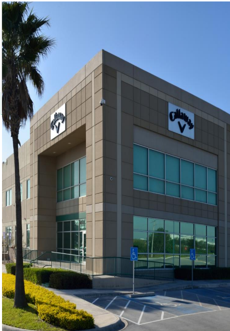
Prologis Apodaca building 2, Monterrey
