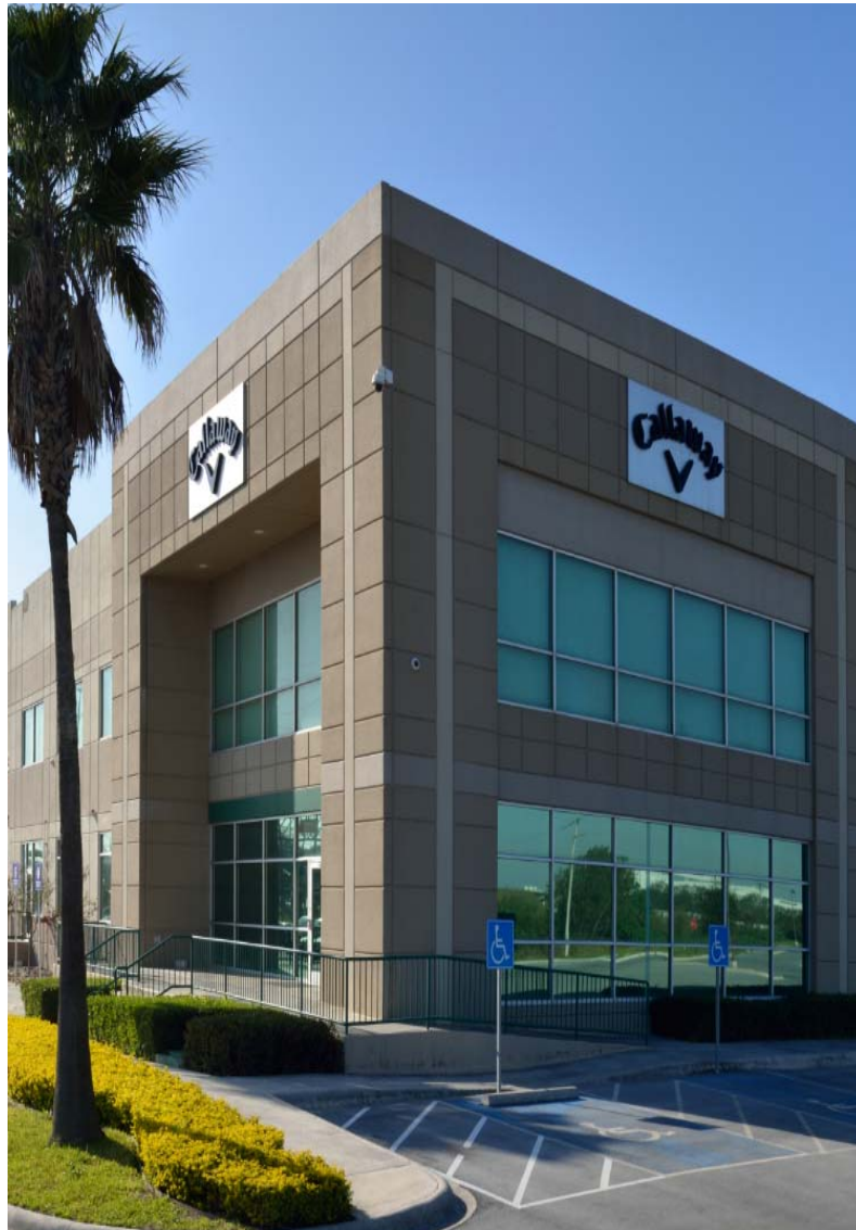
Prologis Apodaca building 2, Monterrey
