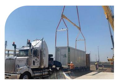
A C1000S microturbine at the Wallumbilla LPG facility is the first gas site in the world to use a butane-fired, grid-connected microturbine to generate power onsite for site electricity demand, while exporting excess power to the grid.
