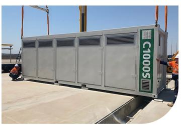
electricity for both operations and gas production. This amounts to roughly 20% of the new system's capacity, so the selection of the C1000 allows AGL to export an excess 800 kW to the grid, which not only benefits consumers, it provides revenue for the company.
