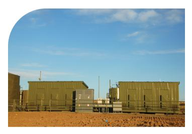
Eight C65 microturbines are fueled by natural gas and run simultaneously to provide power to the remote oil and gas producer located in San Juan Basin, New Mexico.
