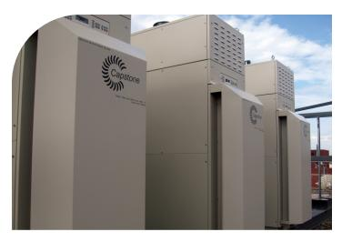
Commissioned in 2019, the rooftop-mounted C65 ICHP microturbines have logged more than 85,000 runtime hours, which amount to 99.8% uptime.
