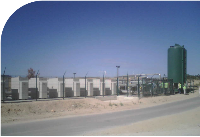
Eighteen C65 microturbines running on methane gas generate power and heat at La Ciotat Landfill in France.
