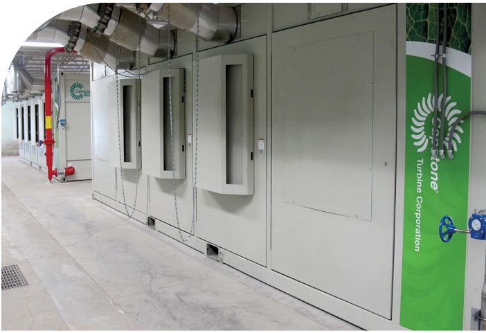
A natural gas and methane gas fueled Capstone C1000 and CR600 at York's wastewater treatment plant save energy, cut operational costs and protect the environment by generating clean-and-green electricity.
