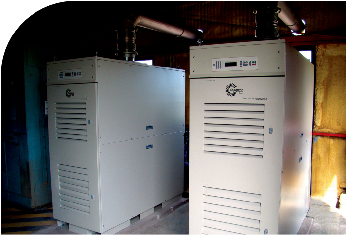
Thirty-five Capstone C65 natural gas-fueled microturbines power compressors at this Bolivian pumping station.
