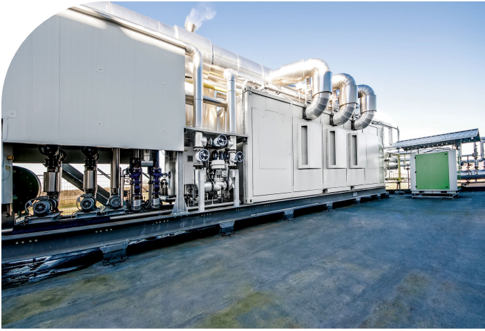
The Capstone C600 system produces heating, cooling and steam for Surgital's new storage warehouse.
