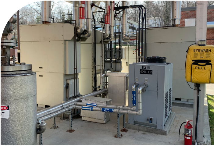
Three C65 microturbines are capable of generating 195 kW covering more than half of the site's total energy use.
