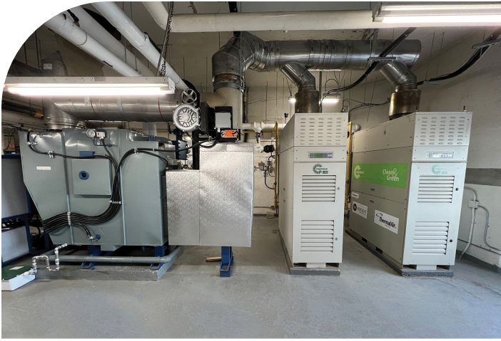
Two C65 ICHP microturbines fueled by natural gas provides 400 McLevin, located in Scarborough, Ontario, reliable power while also reducing energy costs.
