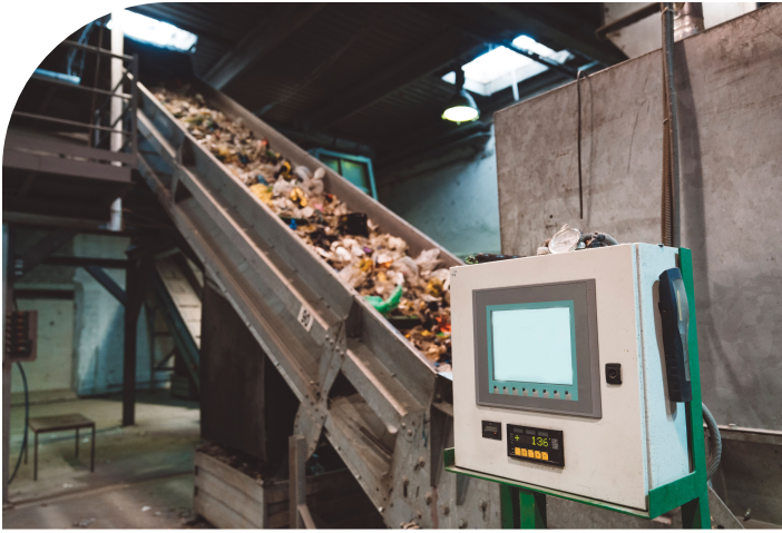
One C800S microturbine converts methane gas collected at the Burbank landfill into clean, reliable and cost effective power.
