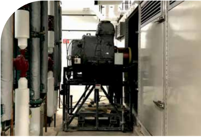
A 1MW microturbine system at Oneida County Water Pollution Control Plant uses the methane byproduct of the digestion process to reduce energy consumption, lower utility costs, and lower environmental impact.
