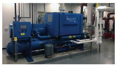
Tecogen is expanding its reach into the indoor agriculture industry, and more specifically cannabis. The company's Techochill's cooling helps remove the heat generated by the thousands of lights that are needed to grow the crops, while the recovered waste heat can be utilized to dehumidify the air. Tecochill units are powered by TecoDrive 7400 engines, which are industrial versions of the GM Mark V 7.4L V8, modified to Tecogen specifications.
