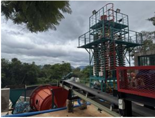
Tivani Toll-milling site in South Africa, showing the spiral concentrator, mill and associated processing infrastructure planned to support demonstration-scale processing of Tivani material
