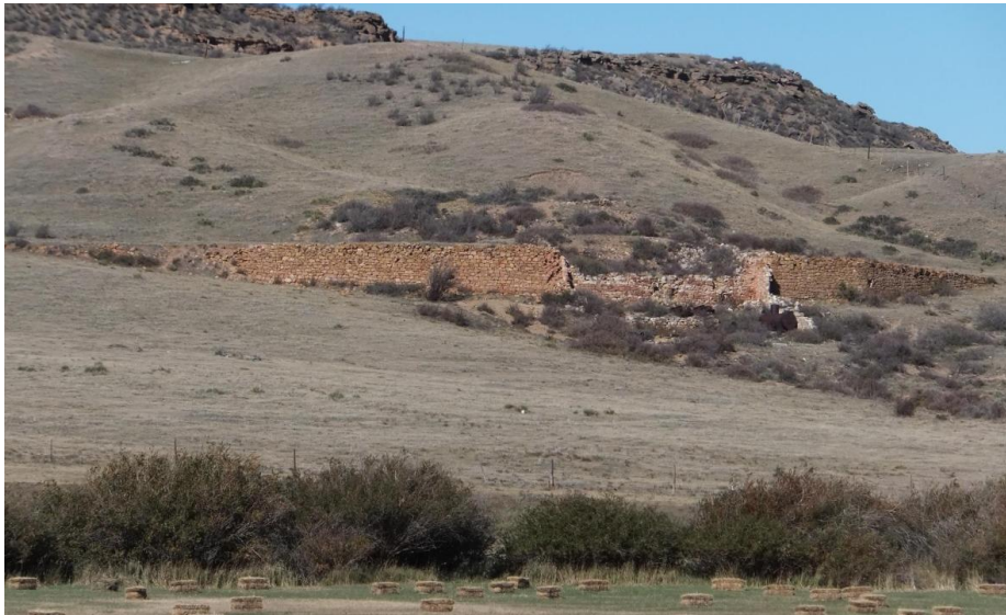
Figure 1– Foundation of the Copper King mill viewed from Laramie County 210 looking north.
