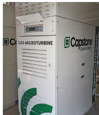
The Winona plant now has two Capstone C65 microturbines that generate electricity and process heat.
