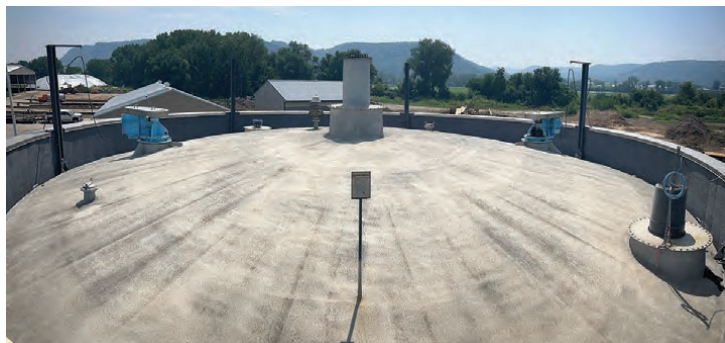
Two blue mixers protrude from the gas cover on one of the digesters at the Winona Wastewater Treatment Plant.
