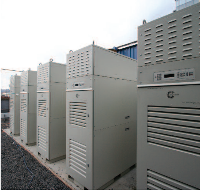
Capstone microturbine CHP plant at Oregon Health & Science University.
