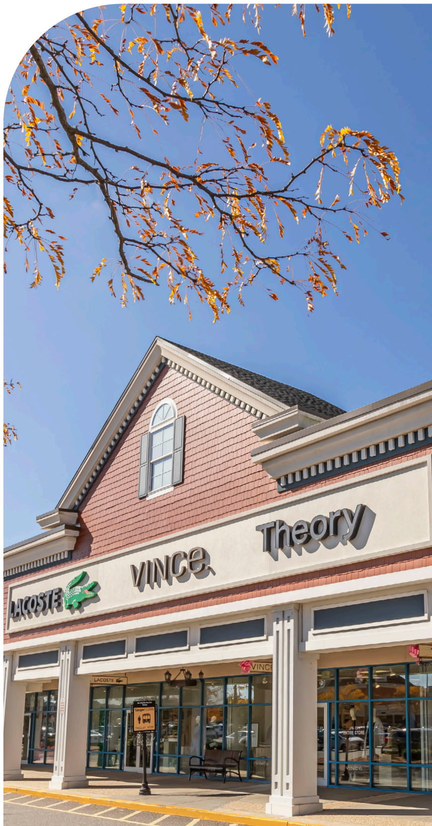
Tanger Outlets Riverhead
