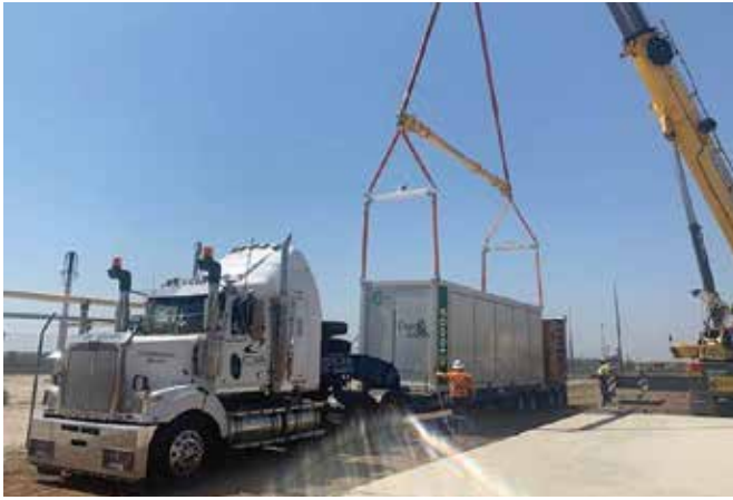
A C1000S microturbine at the Wallumbilla LPG facility is the first gas site in the world to use a butane-fired, grid-connected microturbine to generate power onsite for site electricity demand, while exporting excess power to the grid.
