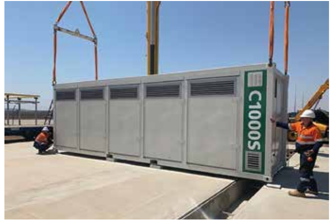
A C1000S microturbine at the Wallumbilla LPG facility is the first gas site in the world to use a butane-fired, grid-connected microturbine to generate power onsite for site electricity demand, while exporting excess power to the grid.
