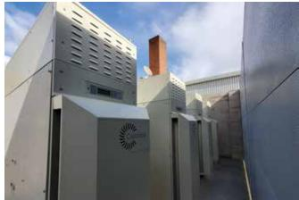
With the installation of four C65 ICHP Capstone microturbines, the Dryden Regional Health Centre has seen a reduction in annual electricity costs of over 50% while powering almost 100% of the hospital all winter and providing 100% of the heating for six months of the year.
