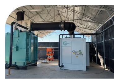
One C1000S Microturbine fueled by liquid natural gas provides the Ascend Growing and Processing Facility in Denver, Colorado with electricity, heating, and cooling while reducing the facility's carbon footprint.
