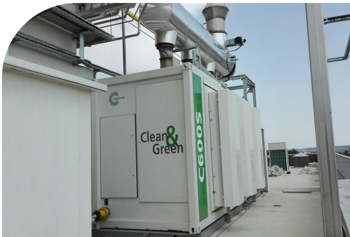
The Capstone C600S Microturbine system utilizes reliable natural gas for Furlotti's processing plant.
