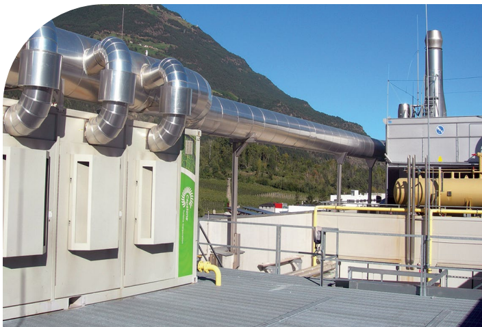
A natural gas C1000 Power Package provides heat and power to the Recla manufacturing plant in northern Italy. Recla produces salami, prosciutto, and other high-end meat products that are exported around the world.
