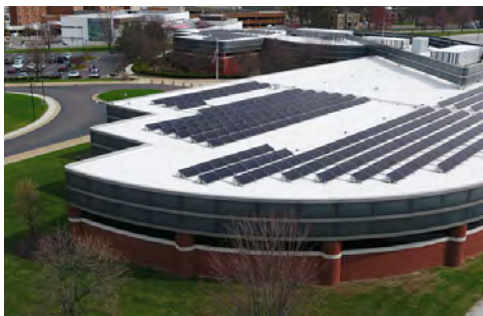
Solar arrays at our Akron facility
