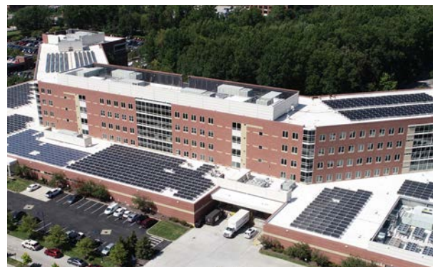
An overhead view of the new solar array at our Easton facility.
