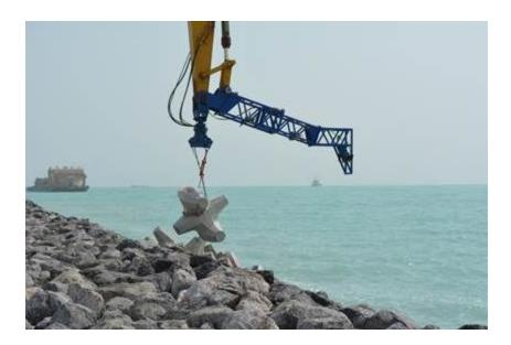
The excavator used for placing the CORE-LOC armour units is equipped with a Coda Octopus Echoscope® 3D imaging sonar providing the operator with real time guidance information during placement below the waterline ensuring the units are placed within the applicable tolerances and according to the rules that need to be adhered to in order to achieve correct interlocking between the separate units.
