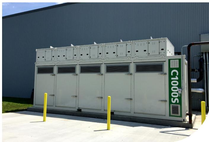
A Capstone C1000S microturbine in a combined heat and power (CHP) application supply the industrial R&D facility's electrical and hot water heating needs.
