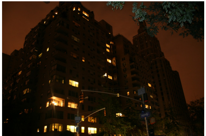
The Brevoort three nights into the Hurricane Sandy blackout with lights shining powered by four Tecogen InVerde CHP units.
