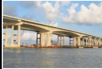
Pelican Island Causeway, Galveston TX
