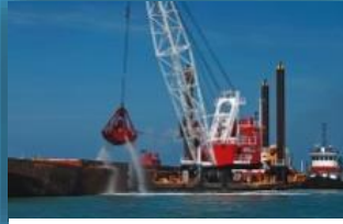
Dredging & Rock Dumping
