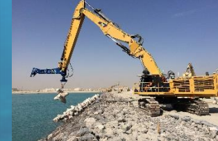
Breakwater Construction
