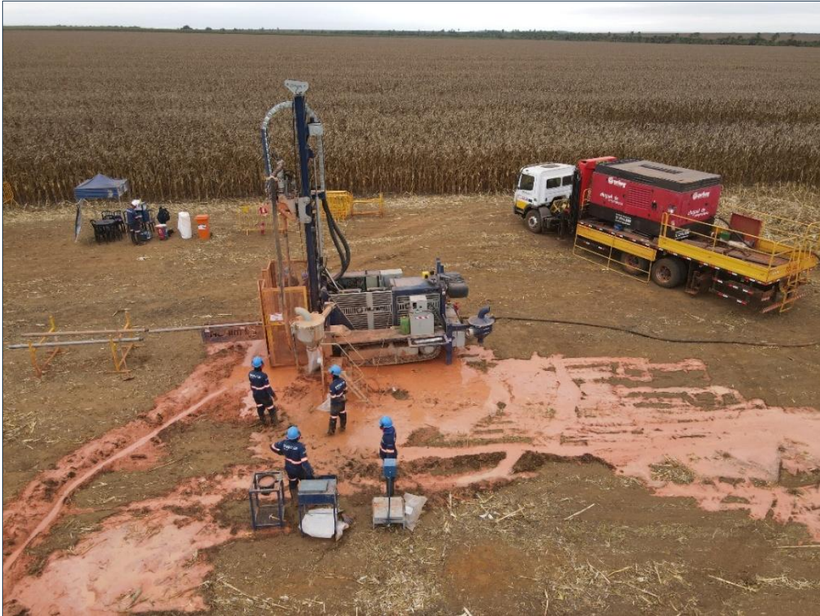
Figure 8: Aerial view of an RC drill rig used during the drilling campaign
