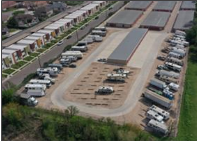
Before / Construction Phase
