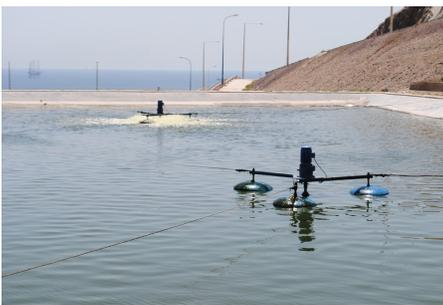
Supplemental aeration with the Moleaer XTB system proved that nanobubbles deliver higher and more stable levels of DO in a warm water environment. It further validated that nanobubbles can enhance an aerobic treatment process and increase the capacity of a system by efficiently reducing the loading.
