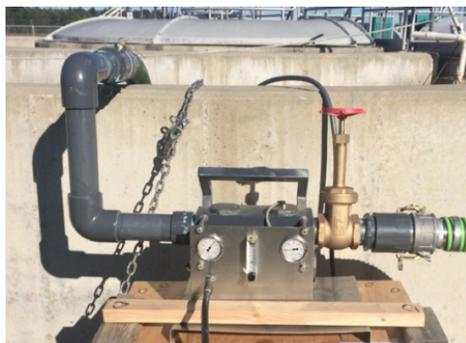
Moleaer 200 XTB installed on the outer ditch of the Village of Warrens (WI) treatment plant.
