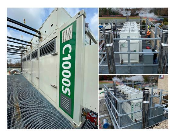
Capstone C1000S Microturbine with Integrated Capstone Heat Recovery Modules
