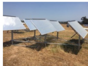
1) Off-the-Shelf Sun-tracking Heliostats (~4 acres per 400 kW)
