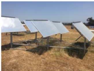
1) Off-the-Shelf Sun-tracking Heliostats (~4 acres per 400 kWe)
