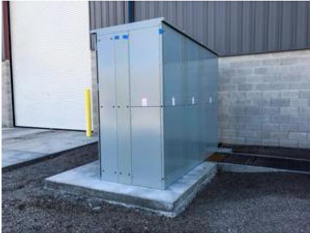
An additional transformer has been installed providing more power to support Phase 1 and Phase 2 electrolyte management projects which includes a membrane filter press, centrifuge and the Phase 2 a dryer that will be used to achieve the remaining 25% of our electrolyte recovery goal.
