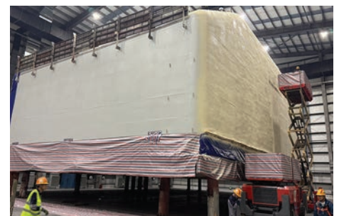
Sections are individually insulated before being joined to form the final, fully insulated tank.
