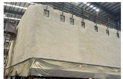
Each complete cargo tank is constructed from four prefabricated quarter sections.
