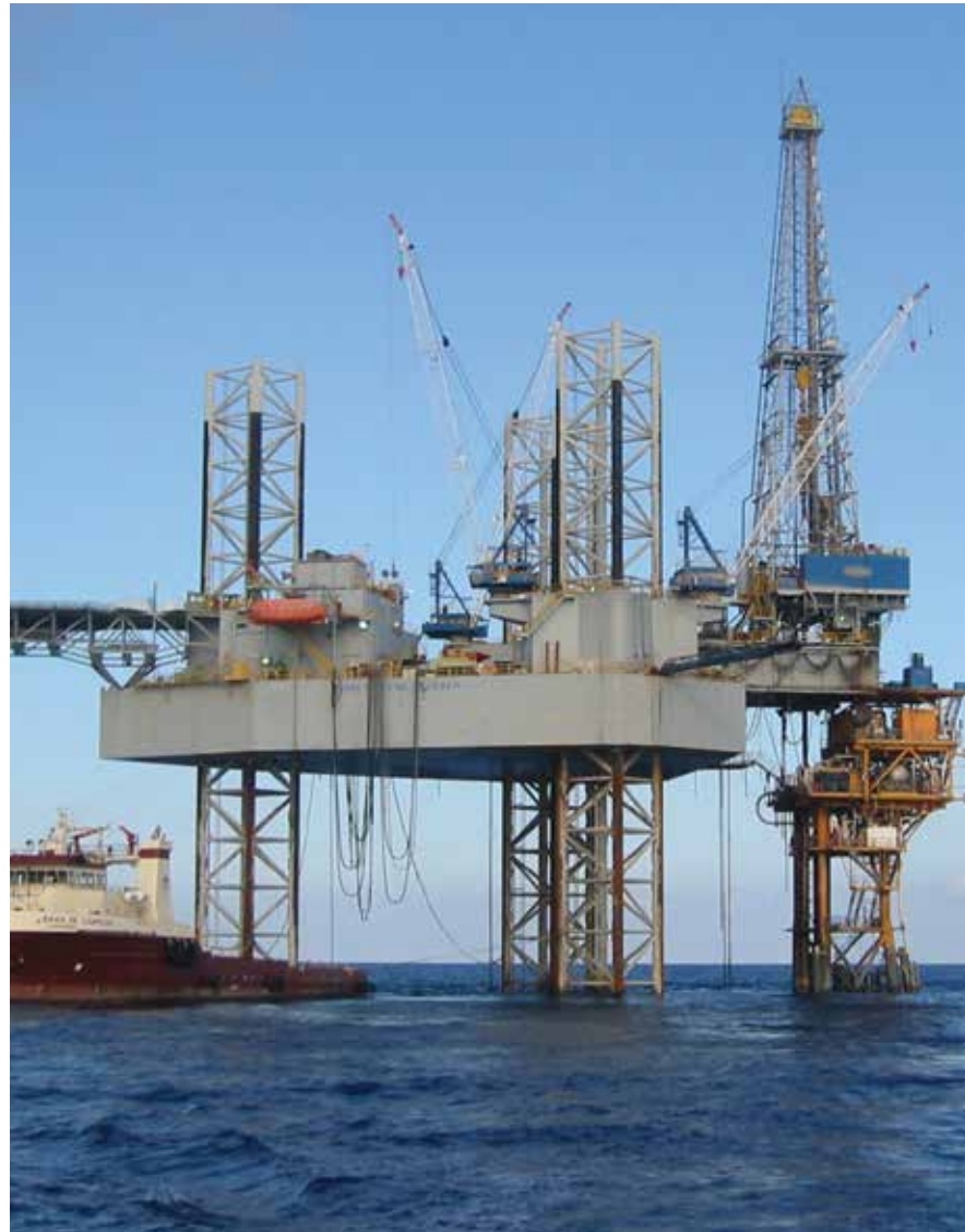
Two Capstone C30, Class I, Division 2 microturbines power this offshore platform in the Gulf of Mexico.
