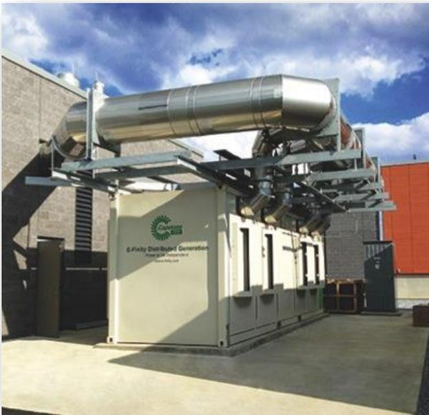
*A Capstone C800 microturbine operating in a CCHP application producing 800kW of clean and reliable power for the PSECU data center UPS, located in Harrisburg, Pennsylvania. Source: Capstone Turbine Corporation*
