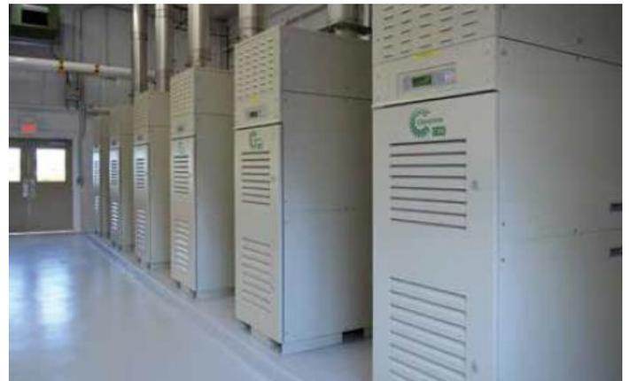
*Natural gas fuels six Capstone C65 Integrated CHP micro-turbines that produce 390kW of clean and reliable power as well as thermal energy for the Viking Yacht Company, located in New Gretna, New Jersey. Source: Capstone Turbine Corporation.*
