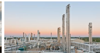
Bridgeport Plant – North Texas
