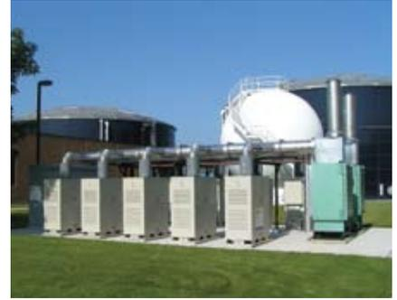
construction and also designed and manufactured the gas treatment system for the biogas. The treatment equipment reduces the moisture level of the gas and eliminates the siloxanes, which are removed using carbon-based filtration media, explains Jan Scott, Unison’s president.
