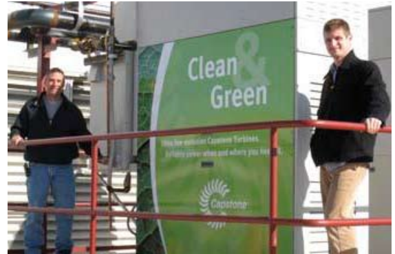
Keystone Redevelopment Group partner Chuck Artillio (left) and project manager Nick Ventresca in front of a new energy efficient system (five Capstone C65 ICHP microturbines sold by Capstone Turbine distributor E-finity) built with stimulus funds.
