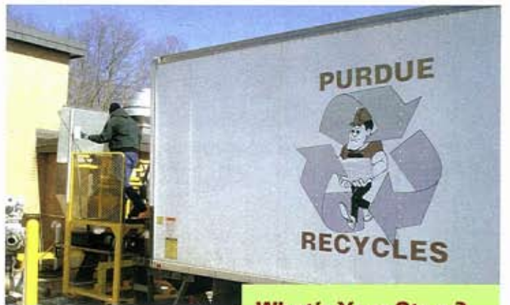
A 35-gallon tote of food waste from Purdue University is dumped into the digester by operator David McKinley at the West Lafayette Wastewater Treatment Plant. The lifting cart was the only expense involved in creating a renewable energy source from what used to be garbage.
