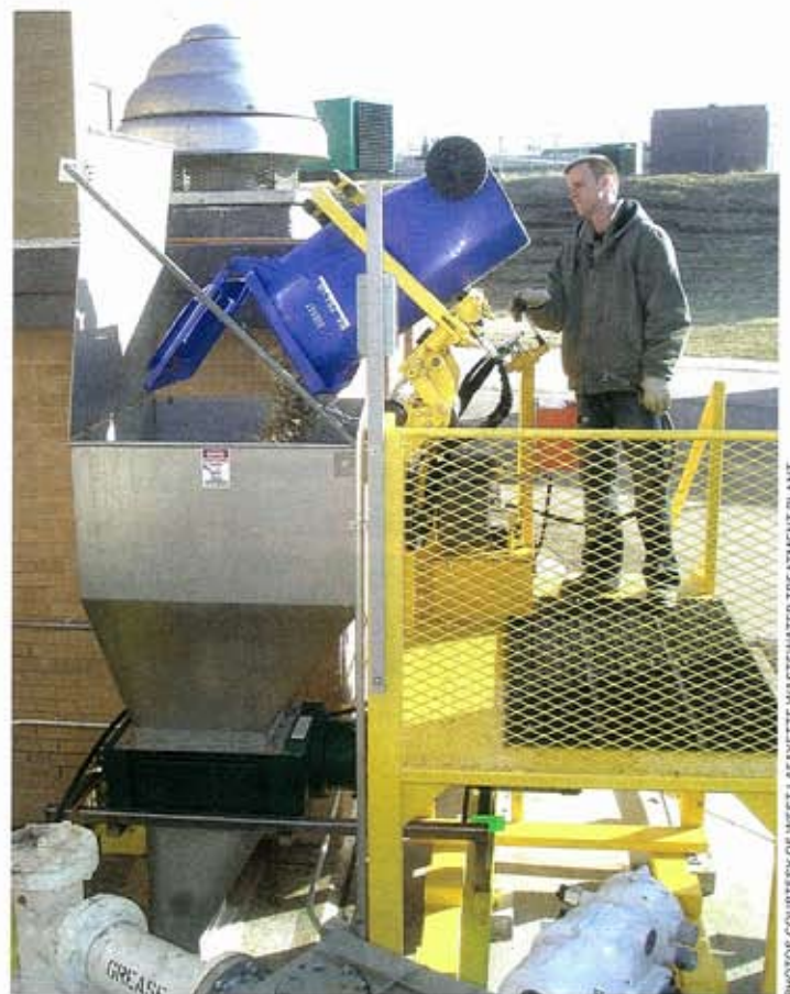
A 35-gallon tote of food waste from Purdue University is dumped into the digester by operator David McKinley at the West Lafayette Wastewater Treatment Plant. The lifting cart was the only expense involved in creating a renewable energy source from what used to be garbage.
