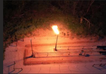
50 MW Flare Gas-to-Power
