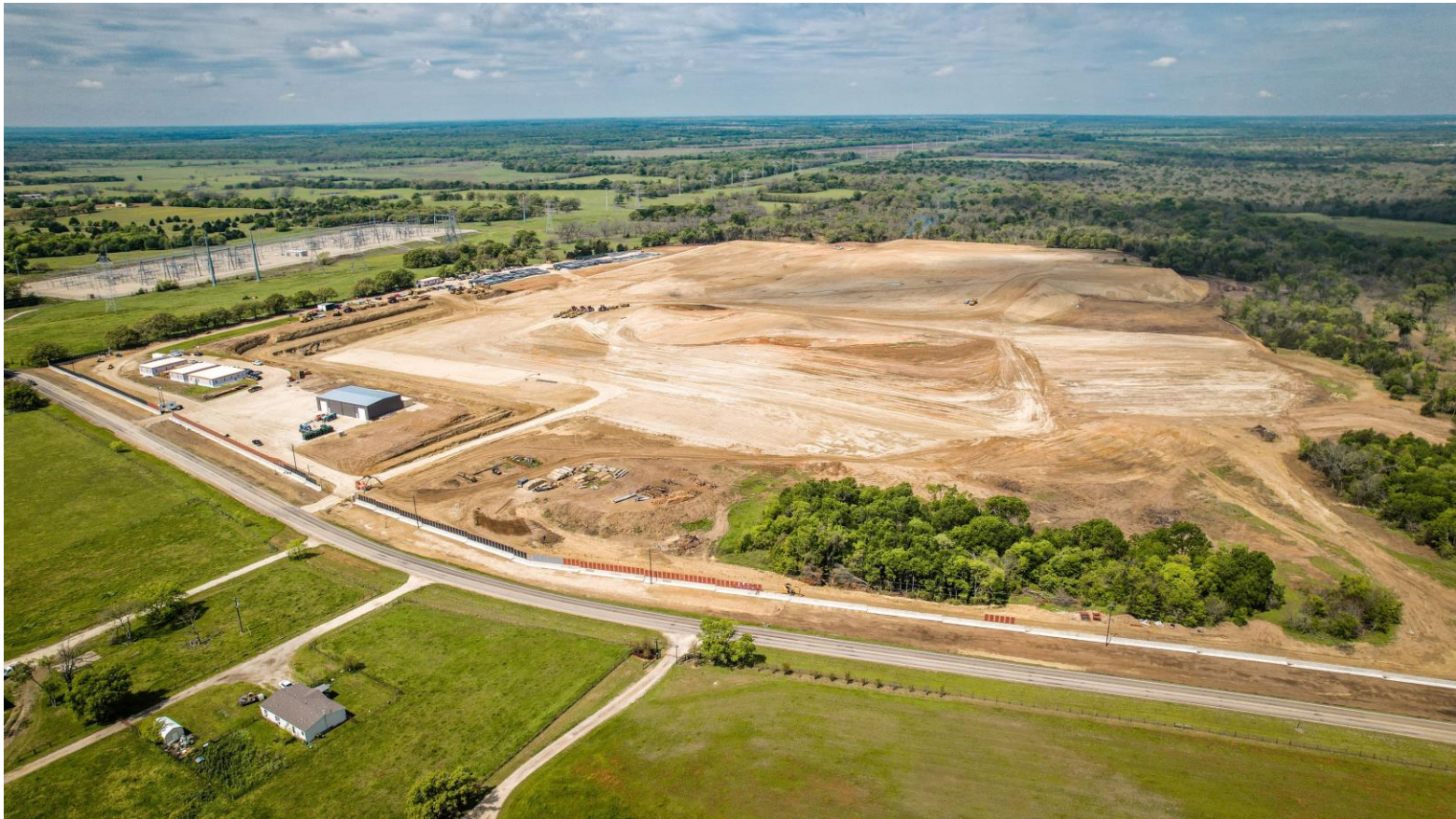
Aerial shot of Corsicana Facility development site
