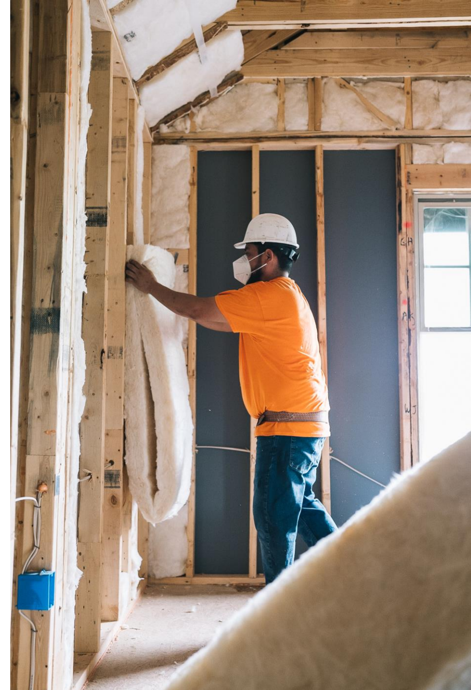
TruTeam residential insulation installation in progress.
