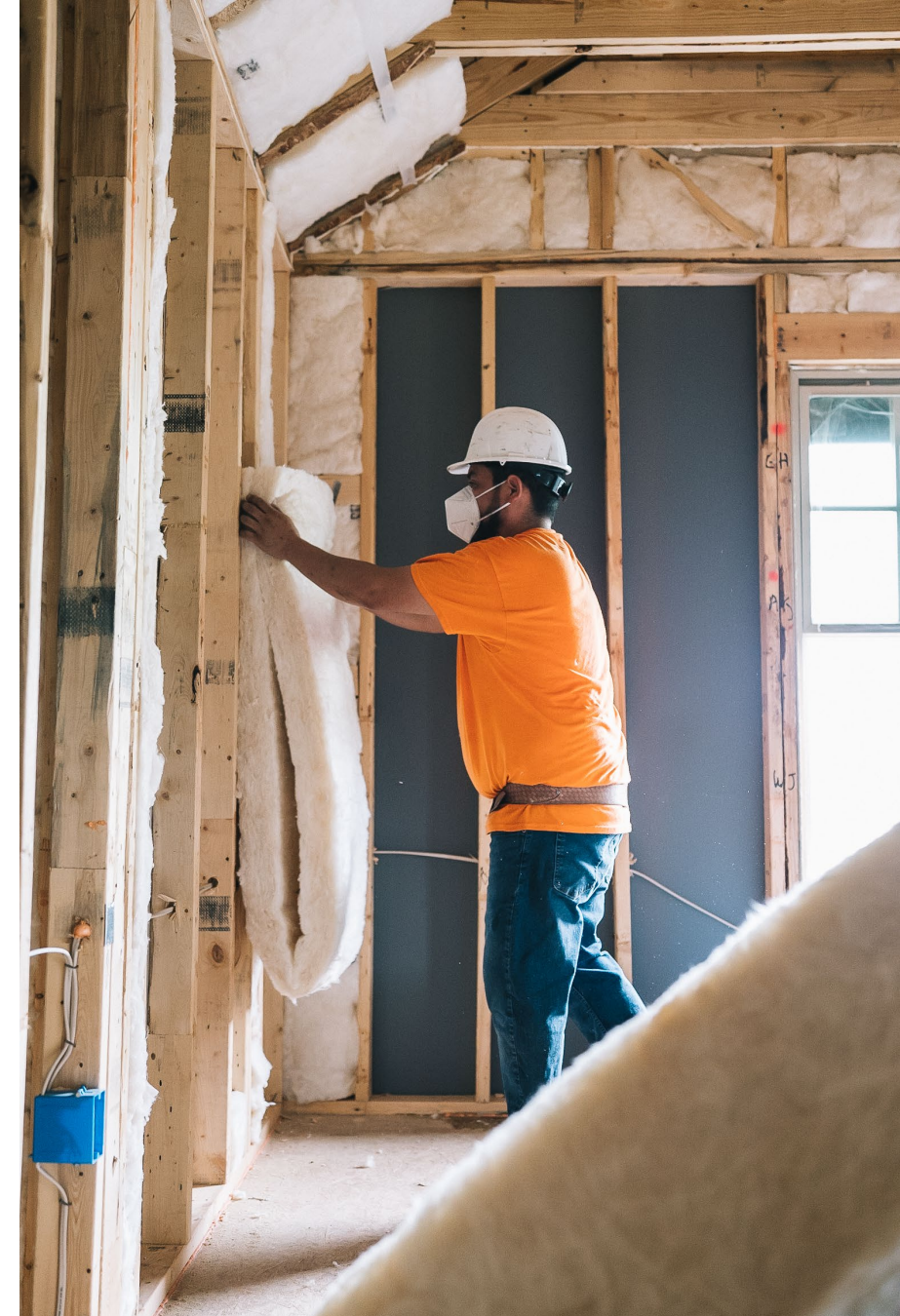
TruTeam residential insulation installation in progress.
