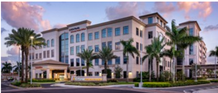
HCA Florida University Medical Office Building – Davie, Florida.
